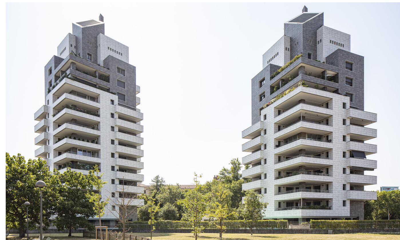
Torre stella - Residential | Milan - Italy V4 fixing system - Visible fixing ventilated façade system for Florim tiles – maximum tile size 80x180 cm - 9 mm thickness
