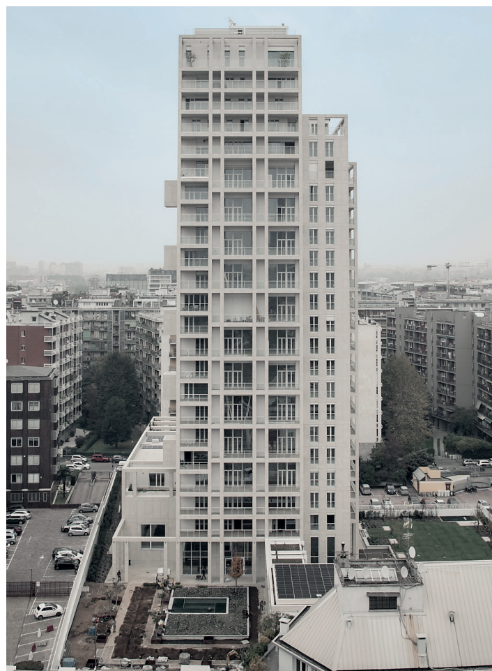
Torre Milano - Residential | Milan - Italy S1 fixing system - Hidden fixing ventilated façade system with FLORIM Magnum slabs – maximum size 160x320 cm - 6 mm thickness
