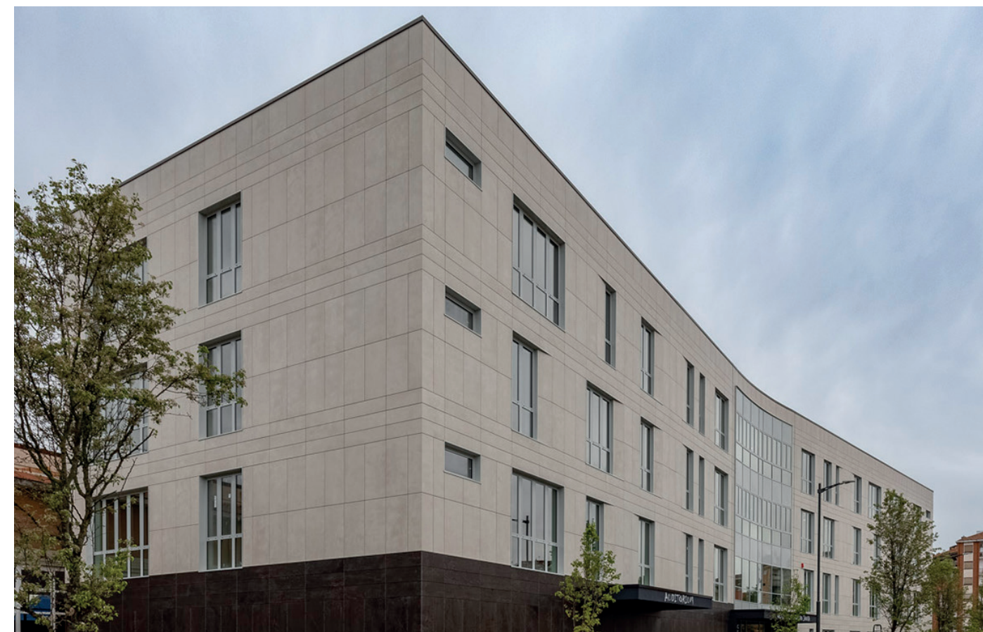
Jona Asti School – Public building | Asti (AT) - Italy V1 fixing system - Visible fixing ventilated façade system for Florim Magnum slabs – maximum size 160x320 cm - 6 mm thickness
